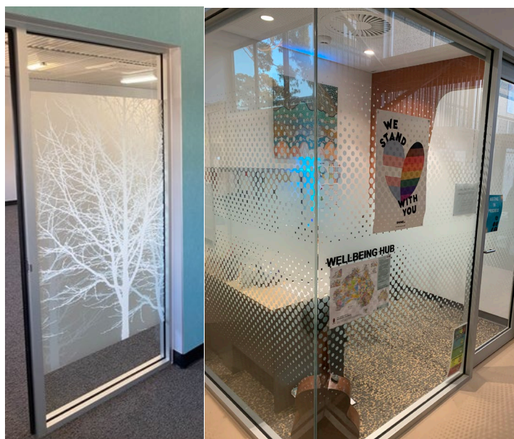
Figure 1: examples of acceptable window glazing providing privacy while still supporting adequate line of sight and supervision.
